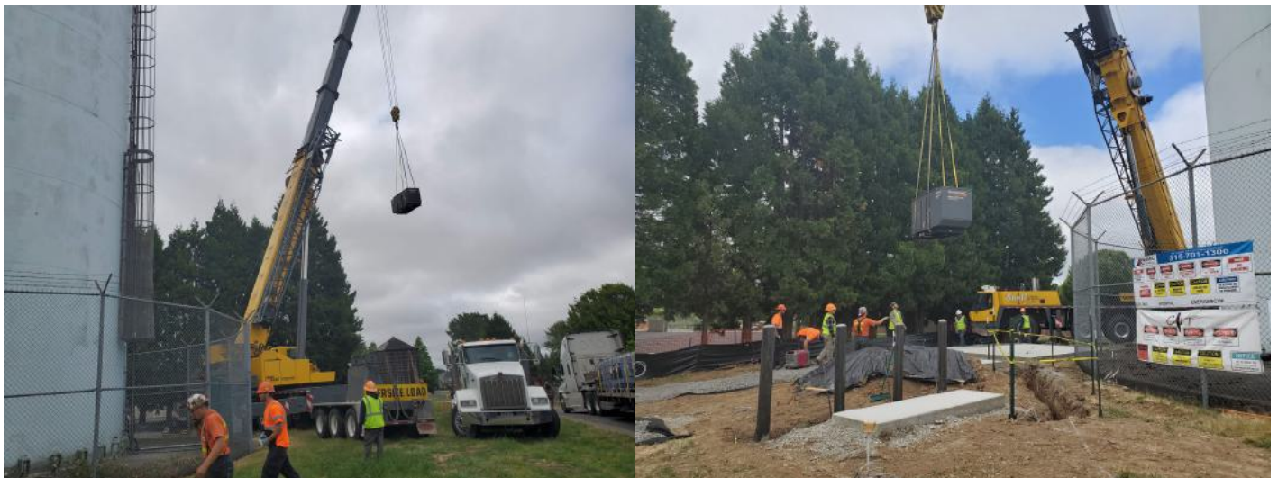
Generator is lifted into place at the new Ridgefield water tower radio site.
